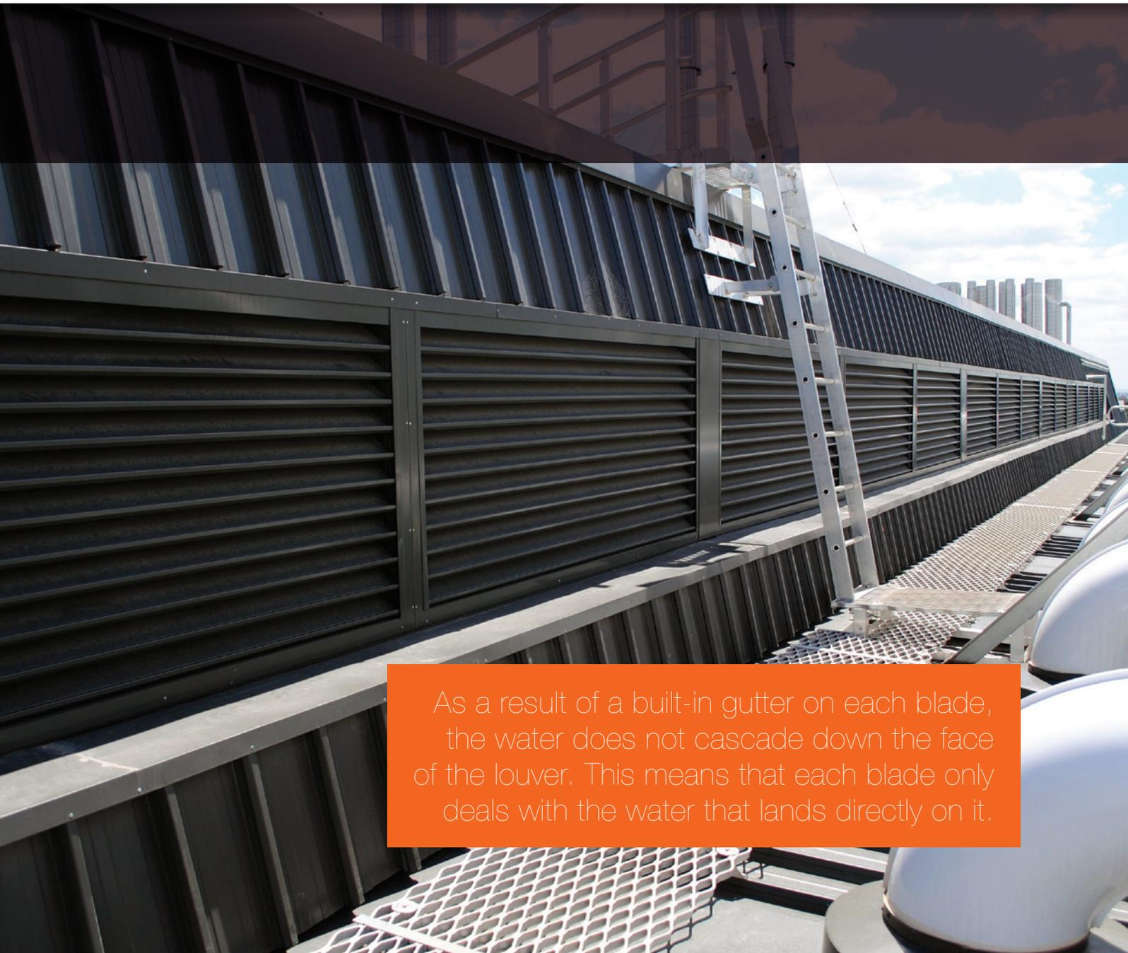
As a result of a built-in gutter on each blade, the water does not cascade down the face of the louver. This means that each blade only deals with the water that lands directly on it.
