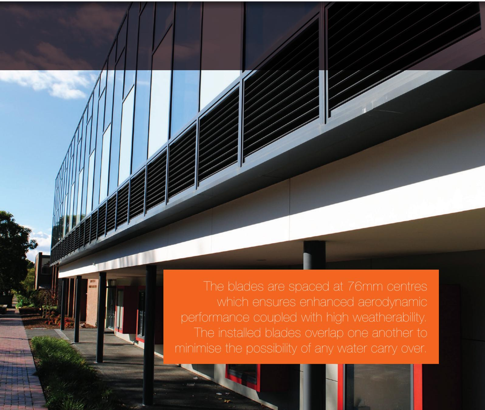
The blades are spaced at 76mm centres which ensures enhanced aerodynamic performance coupled with high weatherability. The installed blades overlap one another to minimise the possibility of any water carry over.
