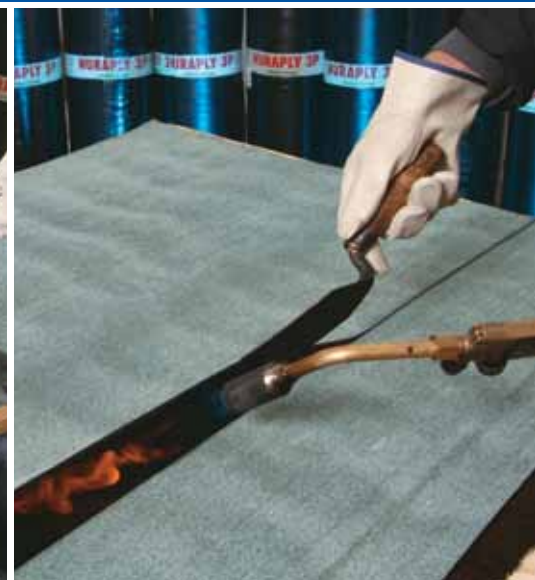
C - Welding lap joints
